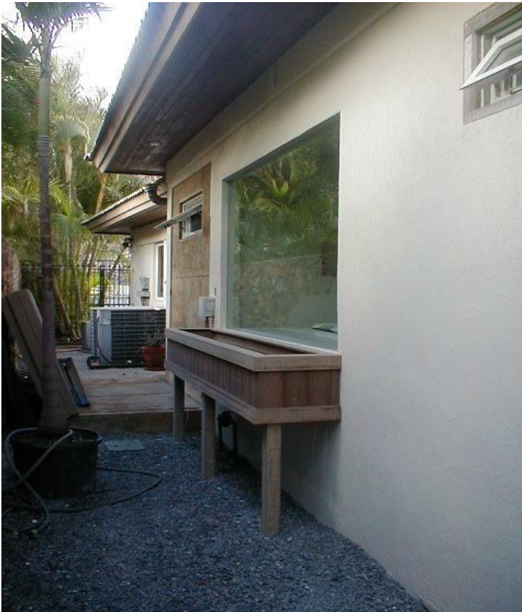
After: Master Suite: Ewa-side wall in progress (looking Mauka)
