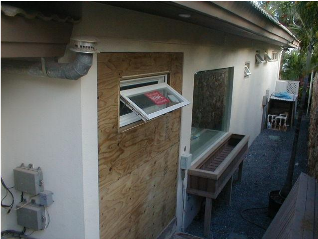
After – Breezeway enclosed
